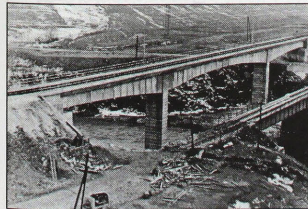
Obr. 5. Most v Margecany tesne po dokončení Fig. 5. Bridge in Margecany immediately after completion
