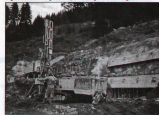
Fig. 2. Anchoring of slope through anchoring beams
