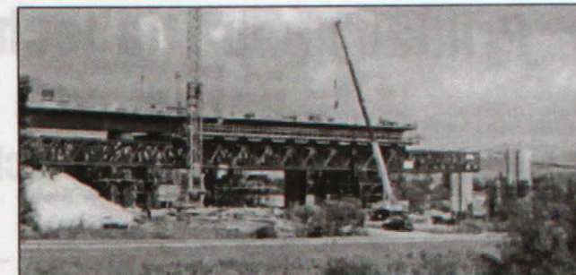
Obr. 4. Pohľad na posuvnú skruž U-40 s debnením ISD NOE Fig. 4. View of the movable centering U-40 with the formwork ISD NOE
