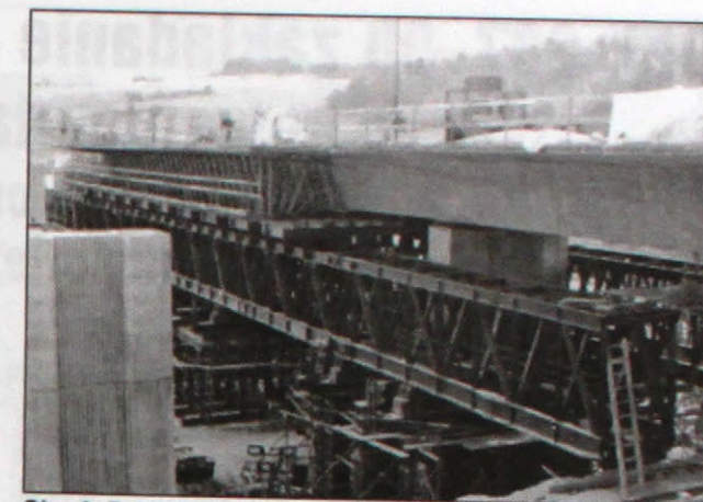
Obr. 3. Pohľad na posuvnú skruž U-40 s debnením ISD NOE Fig. 3. View on the movable centering U-40 with the formwork ISD NOE
