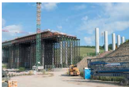
Figure 1: Monitored object (PIŽMO system is the metal supportive construction under the highway deck)
