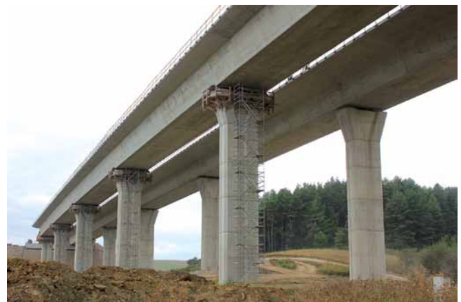
Pohľad na most 205-00 The general view on the bridge
