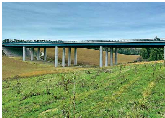
Obr. 8 Hotový most Fig. 8 View of the completed bridge
