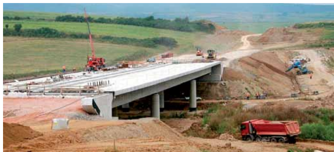
Obr. 8 Most na diaľnici nad potokom Bicír Fig. 8 View of motorway bridge over the brook Bicír
