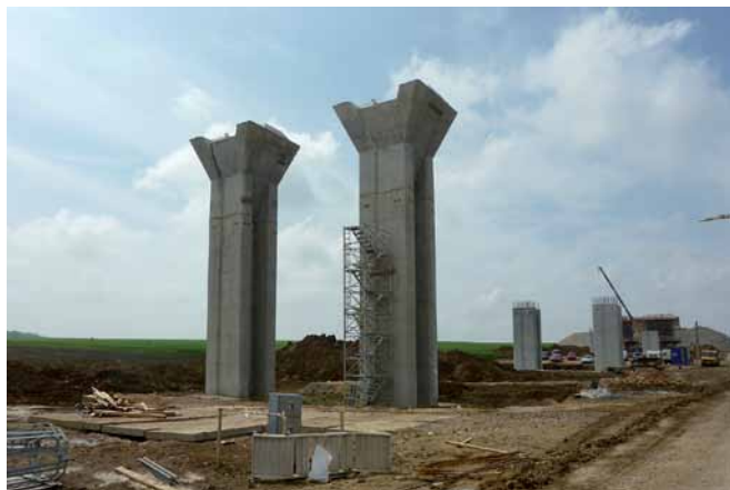
Obr. 3 Budovanie pilierov Fig. 3 Construction of piers
