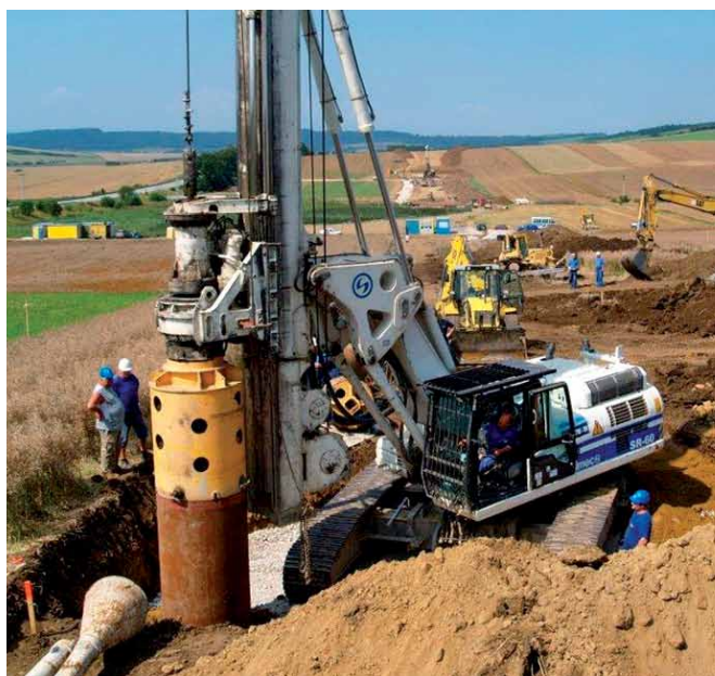
Obr. 1 Zakladanie mosta Fig. 1 Foundation of the bridge
