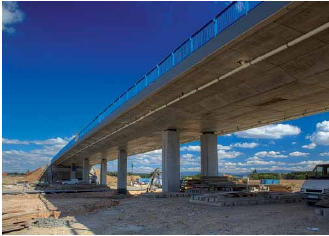
Mostný objekt 201 v križovatke Juh Structure 201 – bridge at the South interchange
