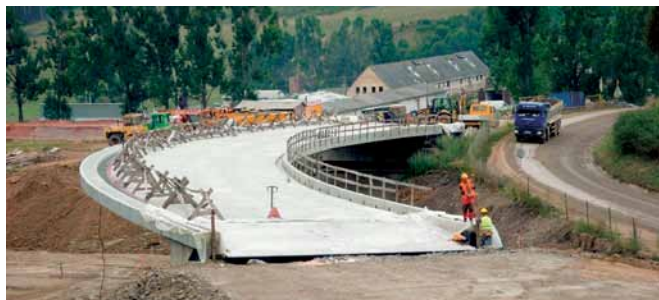
Obr. 7 Most nad diaľnicou na ceste III/18165 Fig. 7 View of bridge on the III/18165 road the motorway
