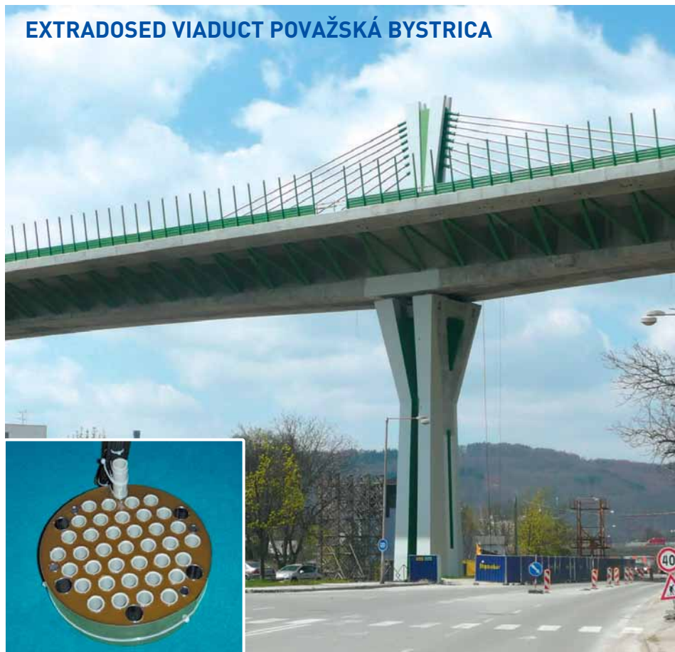
Monitoring of stay cable forces
