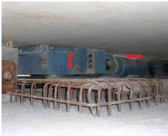
Hydraulické lisy na opore 9, systém zdvihu – posuň Hydraulic presses on abutment no. 9 – "lift-launch" system
