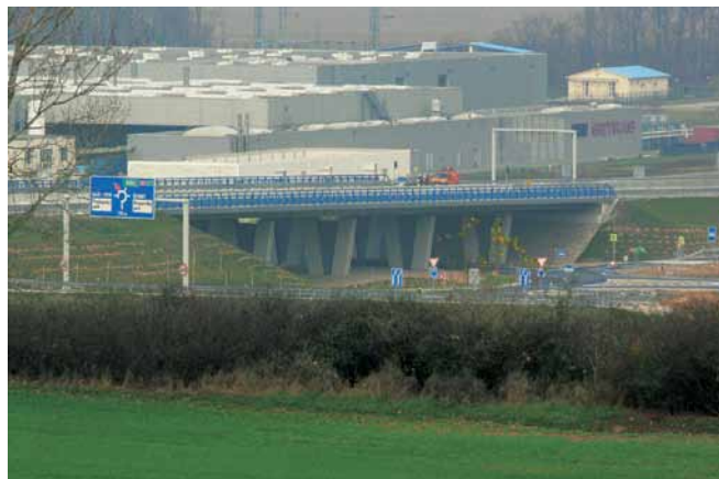
Obr. 3 Most v križovatke Kechnec – SO 215-00 Fig. 3 Bridge at Kechnec crossing – object 215-00
