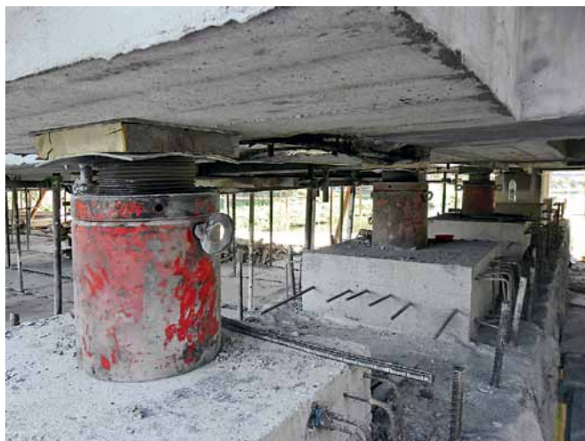
Dočasné podopretie konštrukcie pomocou lisov Temporary support of construction with the usage of presses
