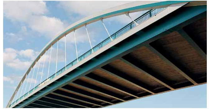
Obr. 4 Oblouk a mostovka Fig. 4 Arch and deck
