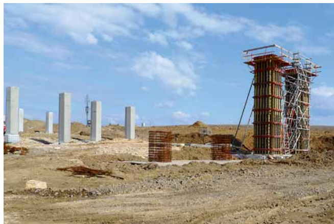
Obr. 3 Stavba pilierov Fig. 3 The pier's construction
