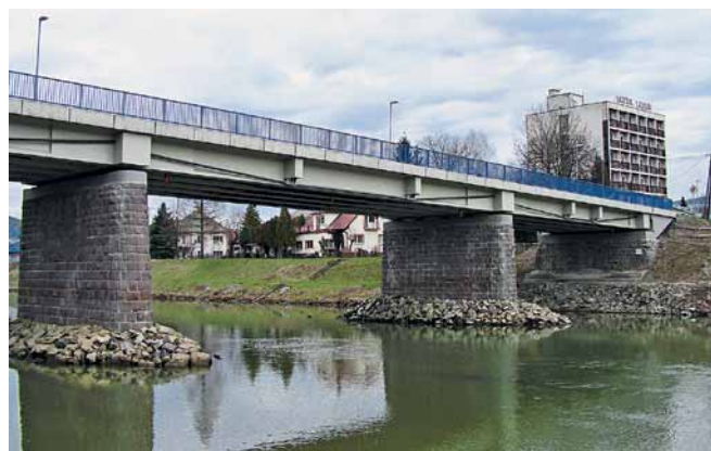
Most po rekonštrukcii Bridge after reconstruction
