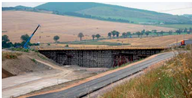
Obr. 3 Most nad diaľnicou na ceste I/18 Fig. 3 View of bridge on the I/18 road over the motorway
