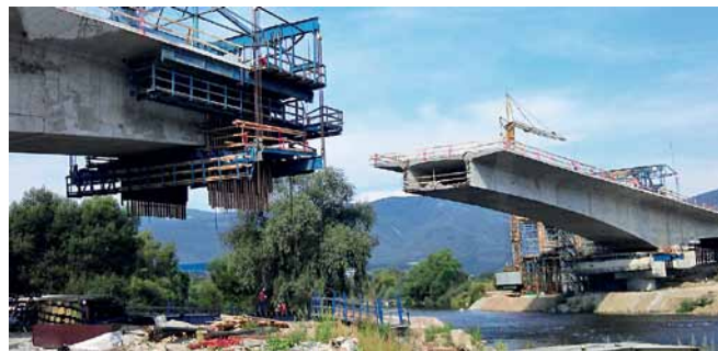
Obr. 7a Budovanie mosta Fig. 7a Realization of the bridge
