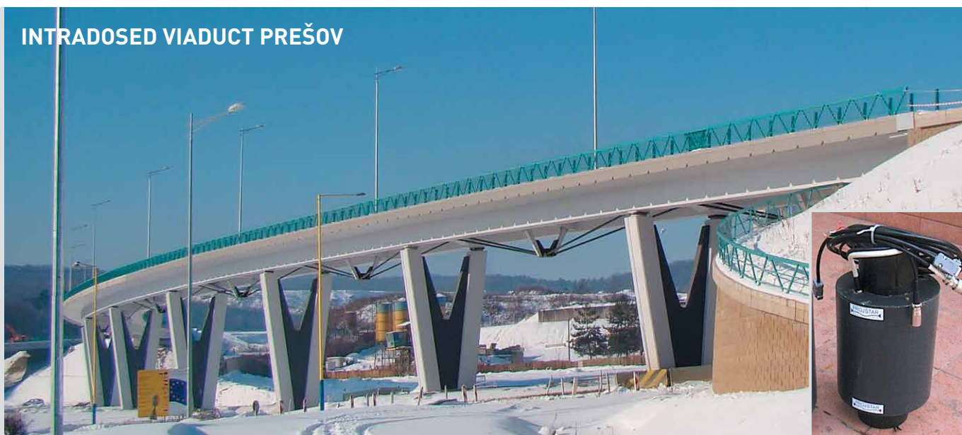
PROJSTAR CH PT system + PROJSTAR PSS Elastomagnetic force monitoring systems for external tendons
