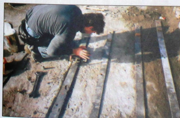
Obr. 5 Zosilnenie mosta pásnicami pri hornom povrchu Fig. 5 Strengthening of bridge by plates installed on the top surface
