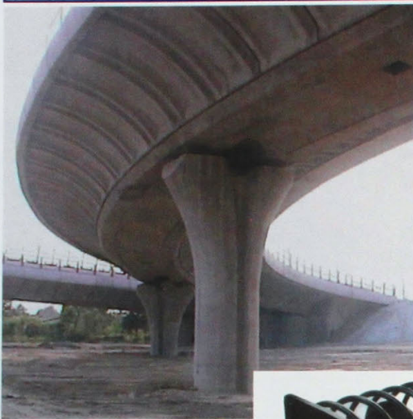
VIADUCT ON HIGHWAY D61 MIEROVÁ-SENECKÁ, BRATISLAVA PROJSTAR CH anchorages
