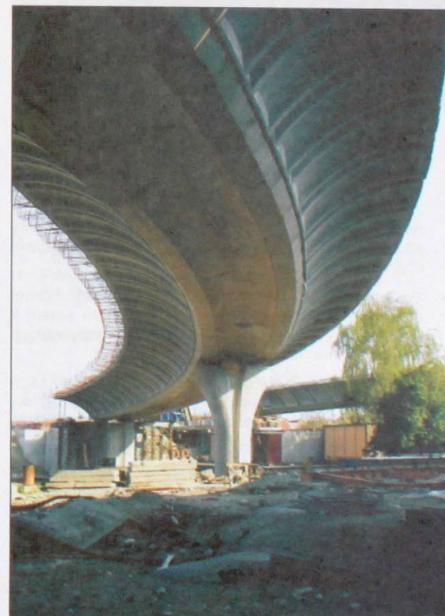
Obr. 6 Most na vetve Fig. 6 The bridge on a ramp
