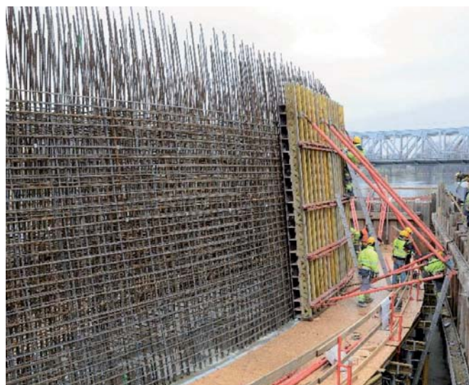
Realizácia piliera Implementation of the pier
