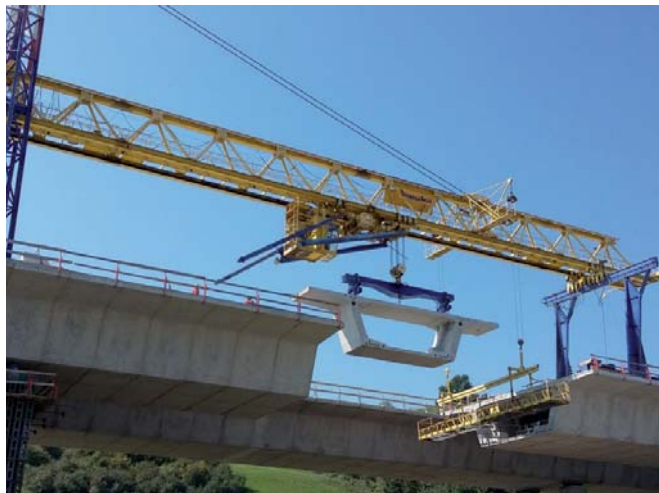
Pohľad na montáž segmentov mosta 209-00 Structure 209-00, view of bridge segments' erection
