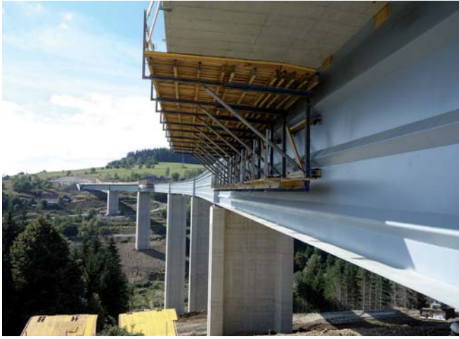
Obr. 1 Debniaci systém Paratop na moste Vřšok Fig. 1 Formwork system Paratop at the bridge Vřšok
