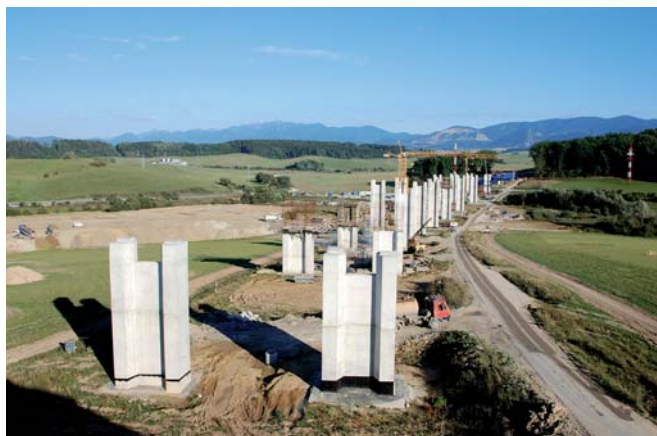
Obr. 2 Pohľad na piliere mosta SO 205-00 v smere na Poprad Fig. 2 View of the bridge piers of the bridge SO 205-00 in direction to Poprad city
