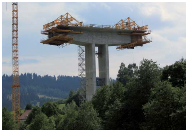
Vahadlo na pilieri P6, budovanie tretej lamely s dĺžkou 5 m Cantilever on pier P6, executing of the 3rd segment with the length 5 m
