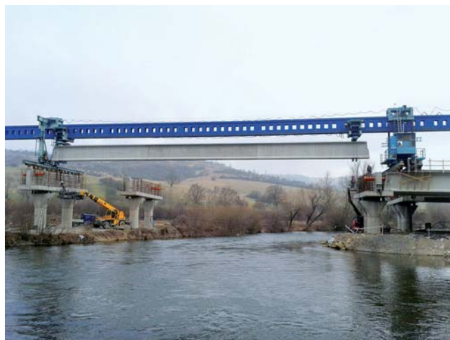
Obr. 7 Ukladanie nosníkov v mieste kríženia s riekou Váh Fig. 7 Laying of beams at the crossing point with the river Váh
