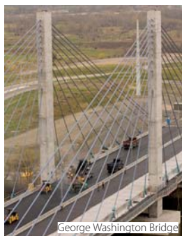
George Washington Bridge
