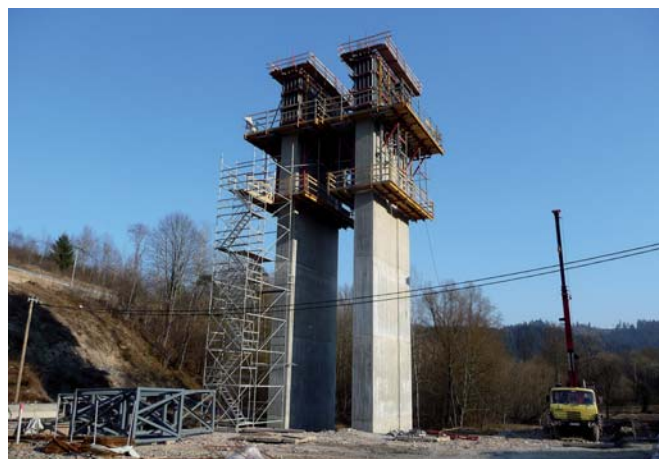
Betonáž stojok piliera P8 pri Markovom potoku po etapách so záberom 5 m Casting of the pier P8 near to Markov stream with stages of 5 m
