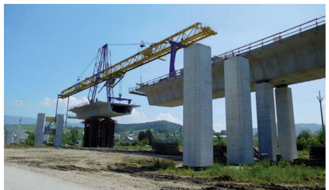
Objekt 209-00, montáž vahadla Structure 209-00, erection of balanced cantilever
