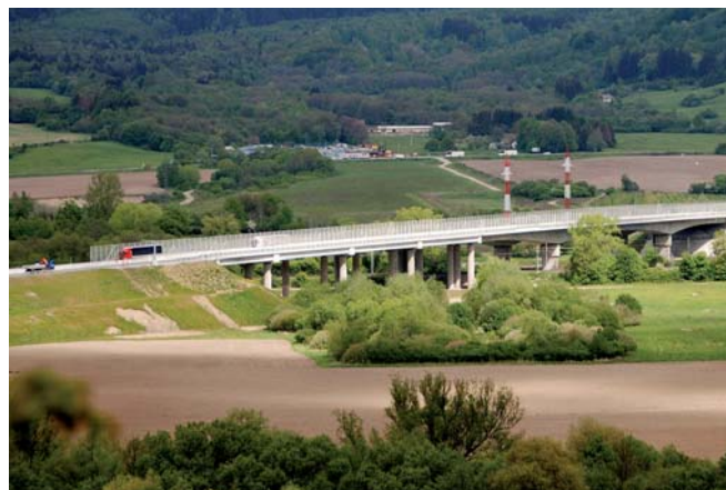
SO 225-00, pohľad na dokončený most Structure 225-00, view of the completed bridge
