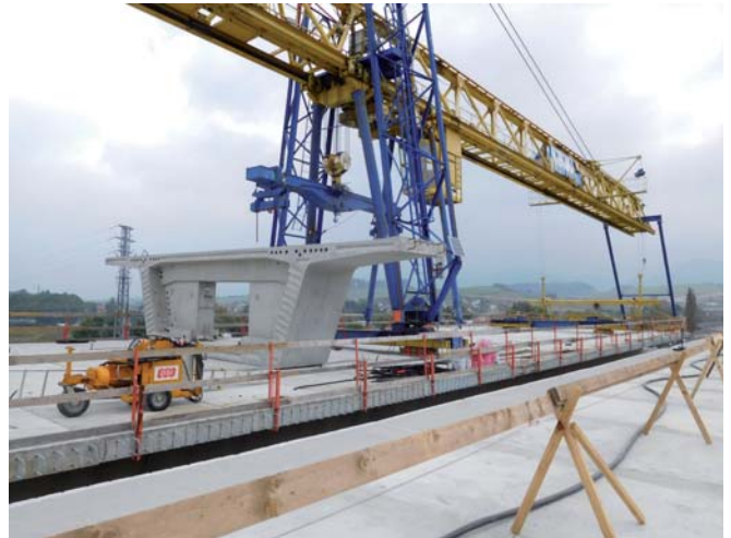
Objekt 209-00, montážne zariadenie a lamela Structure 209-00, the launching gantry and the segment
