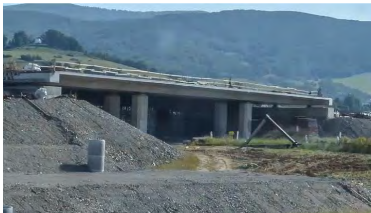
Obr.7 Most na R2 nad III/2632 v km 10.500
