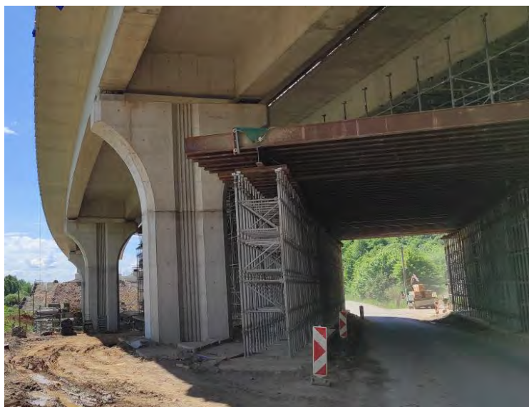
Obr.9 Most na R2 nad III/2664 v km 15.400
